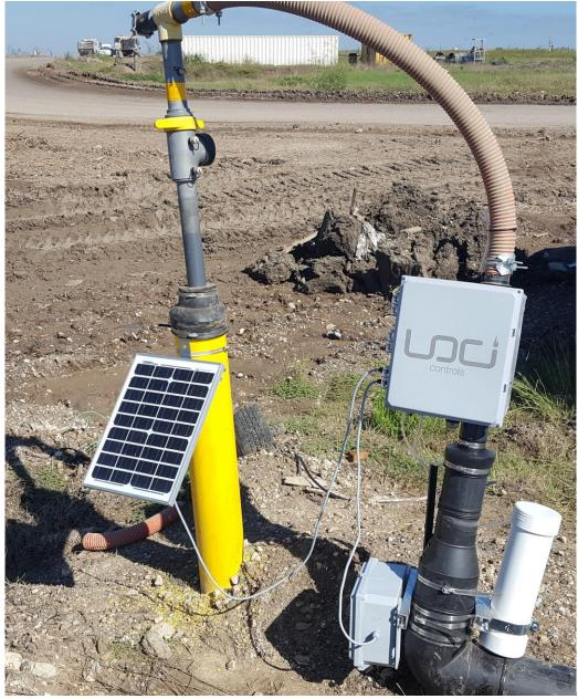
Photo 1: Loci Controller unit on well at the McCommas Bluff landfill in 2018
