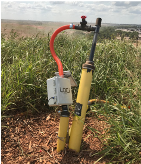
Photo 1: Loci Controller which provides real-time gas composition monitoring and algorithm based well tuning, installed on a gas collector at Oklahoma City Landfill.
